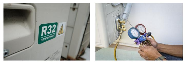
In the normal service life of a heat pump, it should not be necessary to have the refrigerant topped up, but as with all refrigeration systems leaks can develop and repairs by a suitably qualified refrigerant engineer can be needed.
