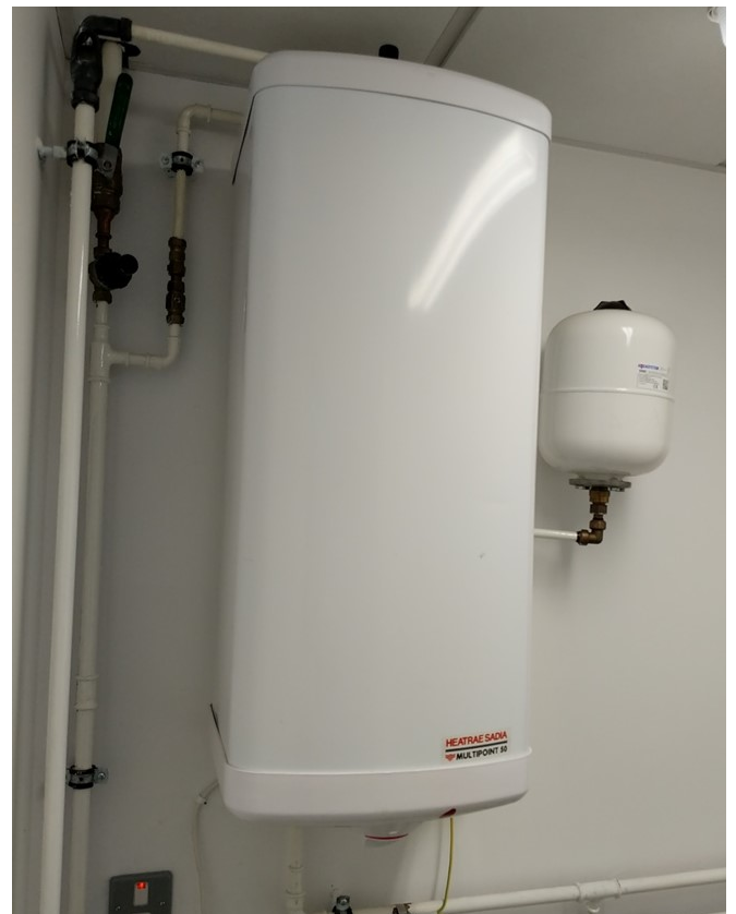
Electric multipoint water heater with integrated storage
